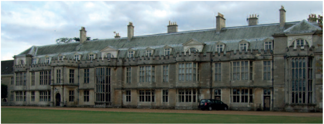
North and South Front, Milton Hall
