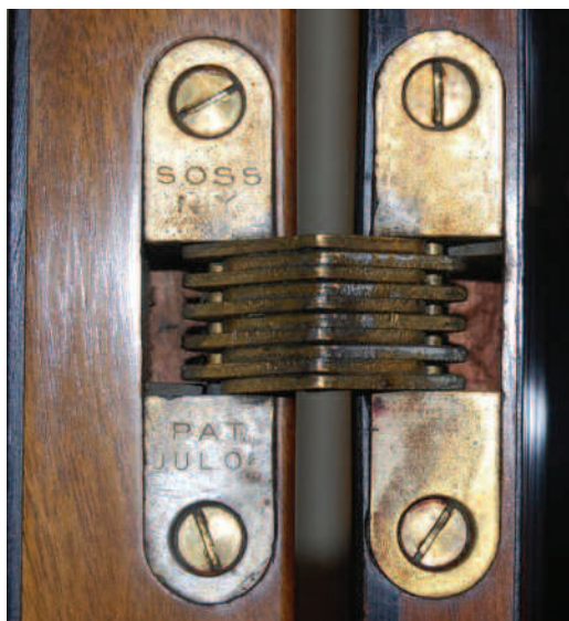
Fig. 7 A SOSS patent hinge fitted on the Duxbury cabinets. Invisible when closed, they prevented catching when dusting
