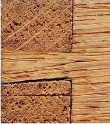
Fig. 2 Detail of wedged dovetail joint on Fiedler commode. By kind permission of the Trustees of the Wallace Collection
